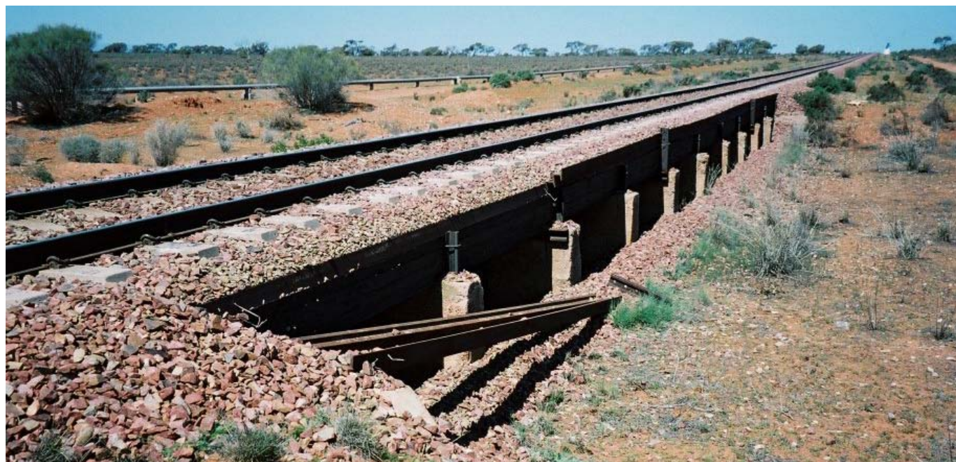
Figure 9 – Consequences of a derailment across a ballast top bridge 14
