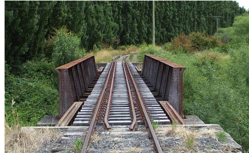
Figure 1 – Guard rail with truncated ends 6
