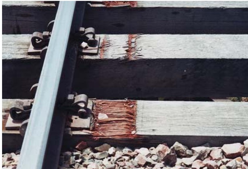
Figure 4 – A guard rail, if provided, could have hindered the passage of a twisted wheelset across this bridge 12
