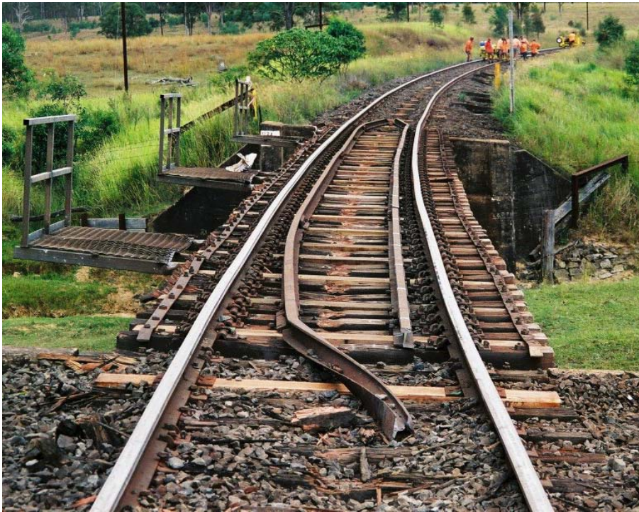
Figure 2 – Guard rails had no effect on behaviour of a derailed bogie 10
