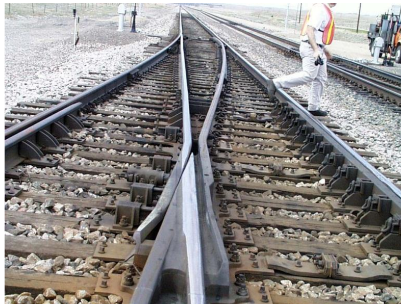
Figure 1 – Spring Wing Crossing ( www.voestalpine.com )
