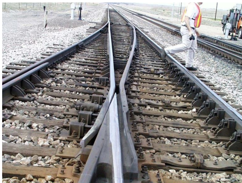
Figure 1 – Spring Wing Crossing ( www.voestalpine.com )
