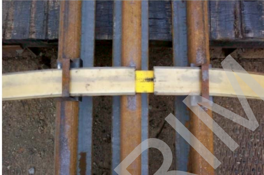
Figure 4 - Webbing, steel cups and nylon sleeves
