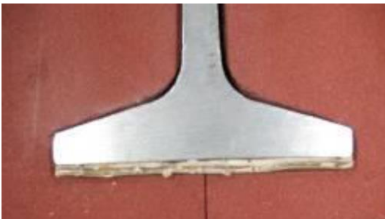
Figure 7: Cardboard filled between weld mould and rail gap (under foot)
