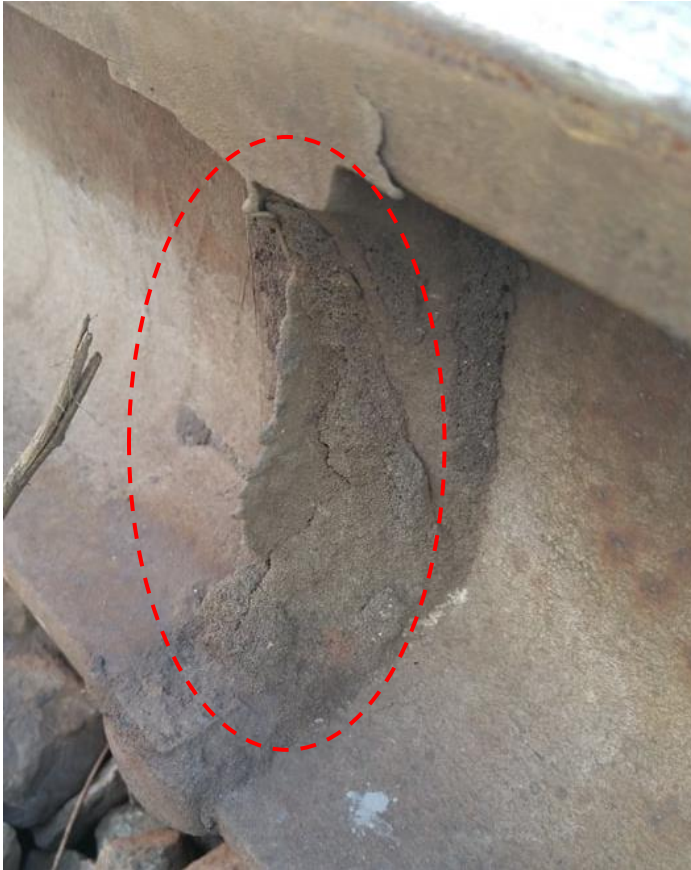
Figure 34: Flashing/finning of the rail weld due to broken weld mould (should be ground off post-weld)
