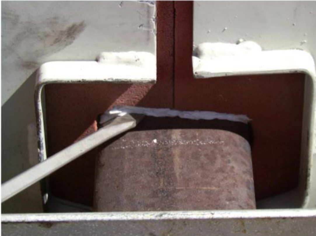
Figure 8: Fit felt between rail head and weld mould if there is a sufficient gap
