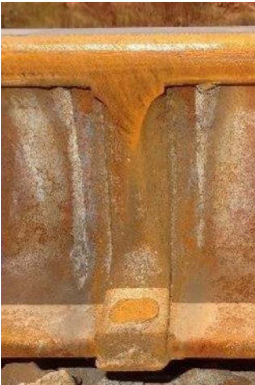
Figure 23: Properly cleaned aluminothermic weld
