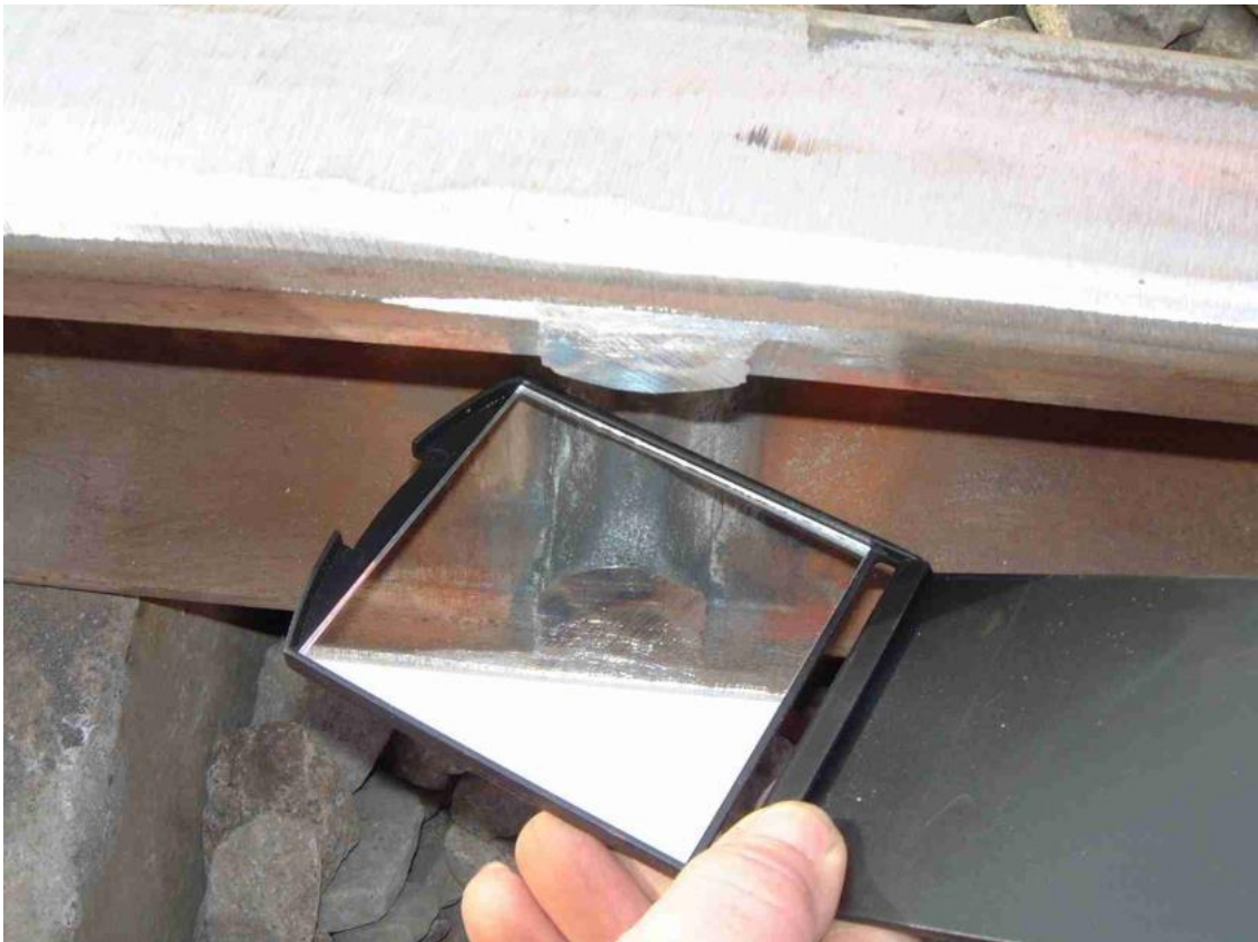
Figure 24: Mirror to check under side of the rail head
