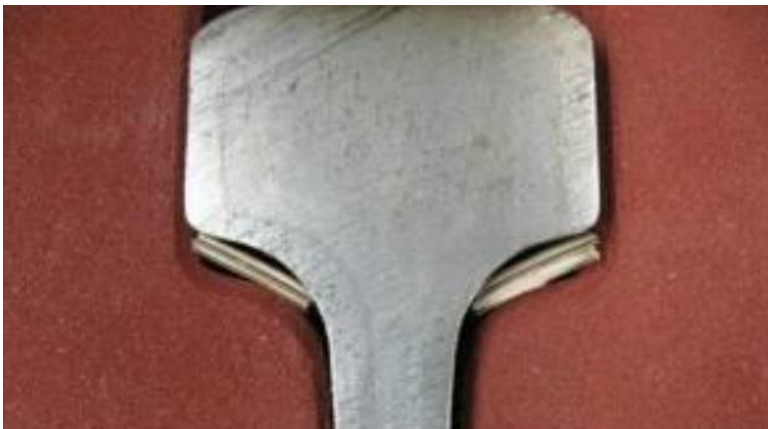
Figure 6: Cardboard filled between weld mould and rail gap (under head)
