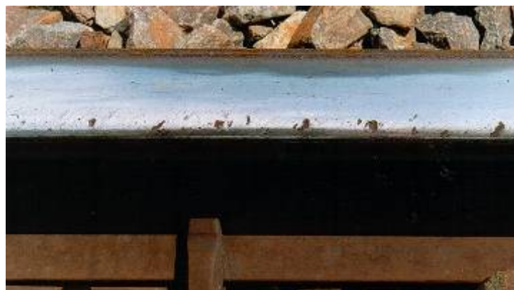
Figure 11(b): Example of Severe Gauge Corner RCF Defects on High Rails Requiring Application of the ARTC H3 Profile
