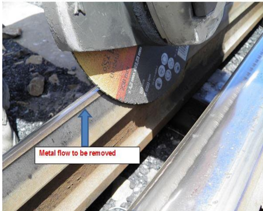
Figure 4-1: Switch blade profiling by grinder
