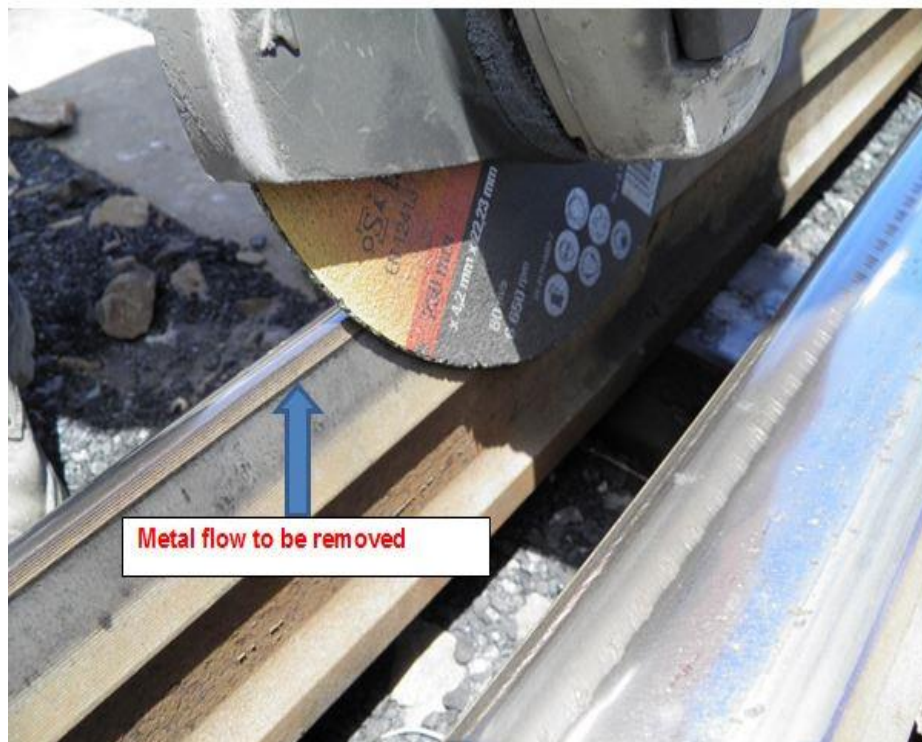
Figure 4-1: Switch blade profiling by grinder
