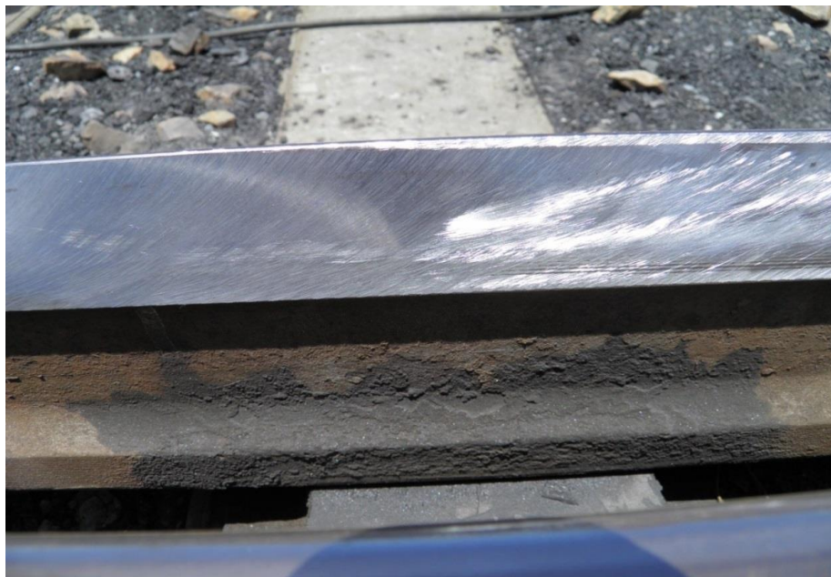
Figure 4-2: Completed profile of the switch blade
