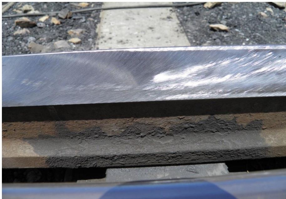
Figure 4-2: Completed profile of the switch blade
