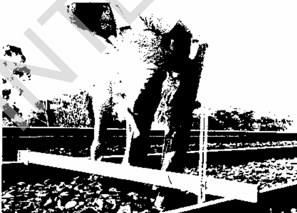
Figure 4 - Measuring Superelevation
