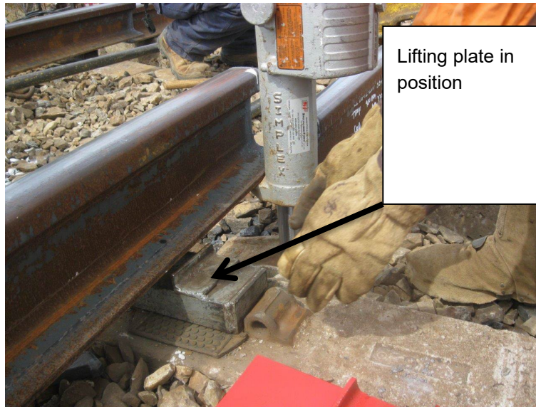
Figure 5 - Insert rail lifting plate (required for overlapping rail ends)
