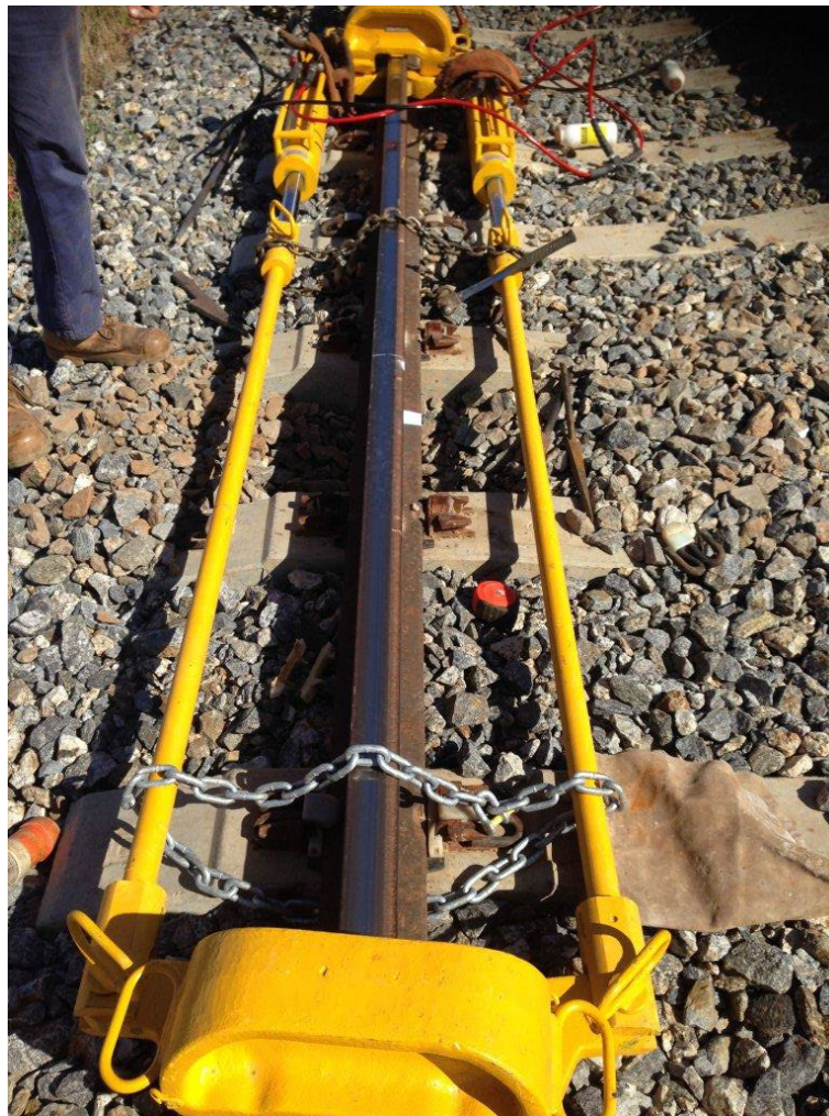
Figure 4 - Tensor setup. Ensure that safety chains are firmly connected to tensor arms under rail foot. Remove slack from restraining chain.
