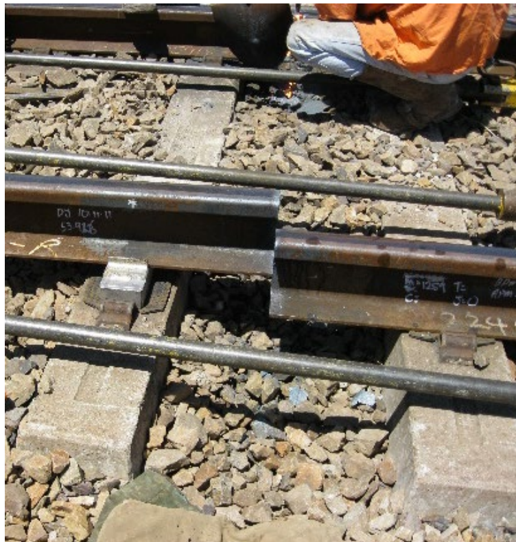
Figure 6 - Rail extension and relaxation process
