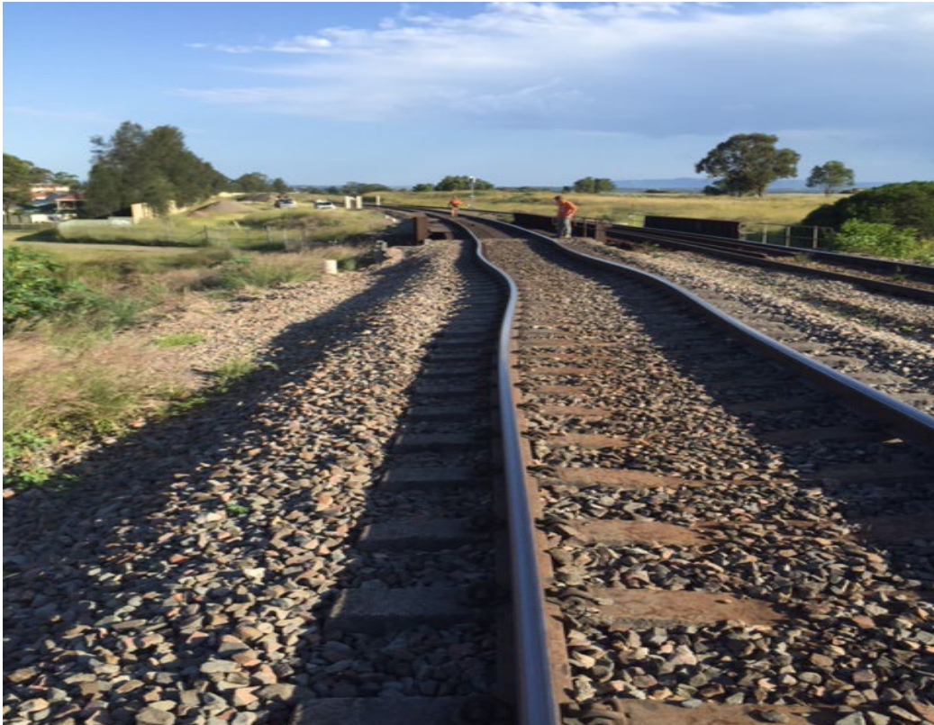
Figure D3 - Example Site 3 Photograph
