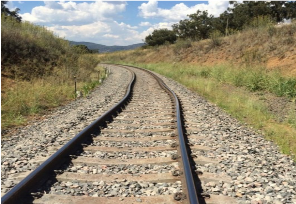
Figure D2 - Example Site 2 Photograph
