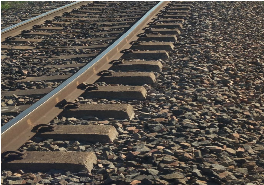
Figure C2 - Ballast profile at the location of the buckle
