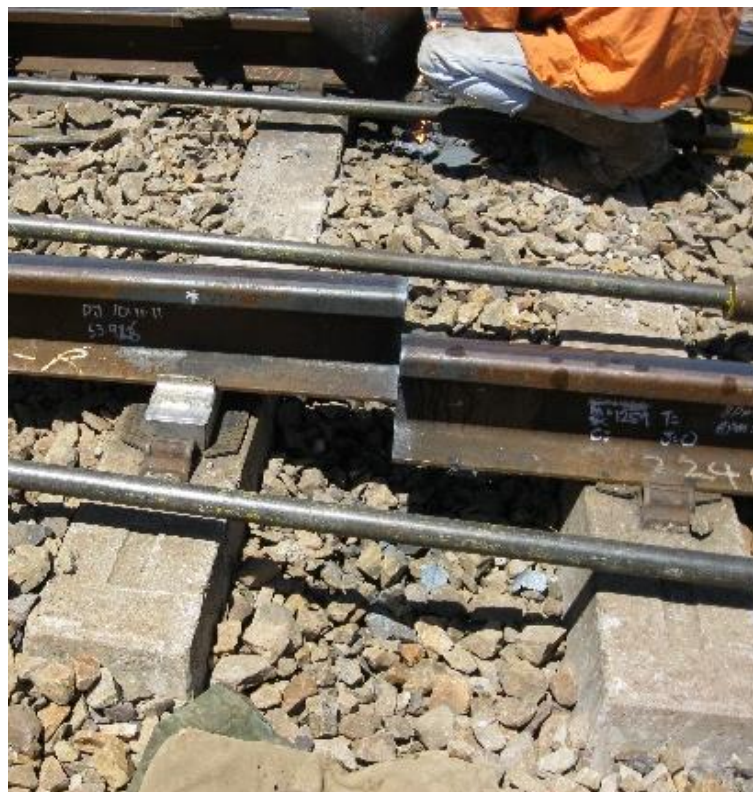
Figure 6 - Rail extension and relaxation process
