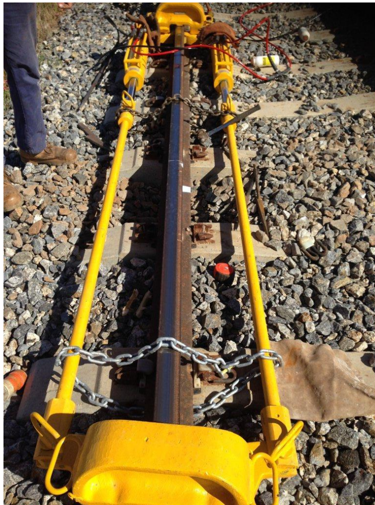
Figure 4 - Tensor setup. Ensure that safety chains are firmly connected to tensor arms under rail foot. Remove slack from restraining chain.
