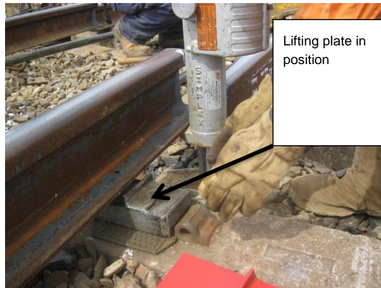
Figure 5 - Insert rail lifting plate (required for overlapping rail ends)
