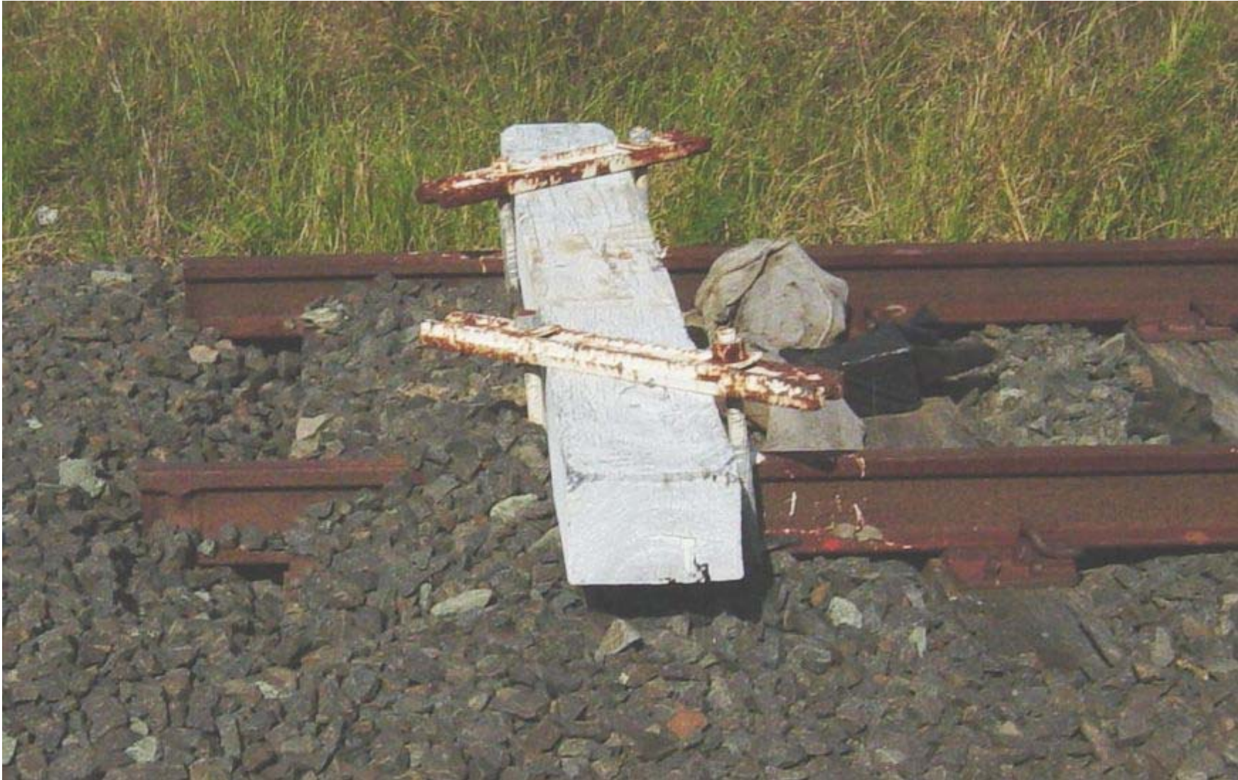
Figure 3 – Photo of ARTC Maintenance Siding Buffer Stop
