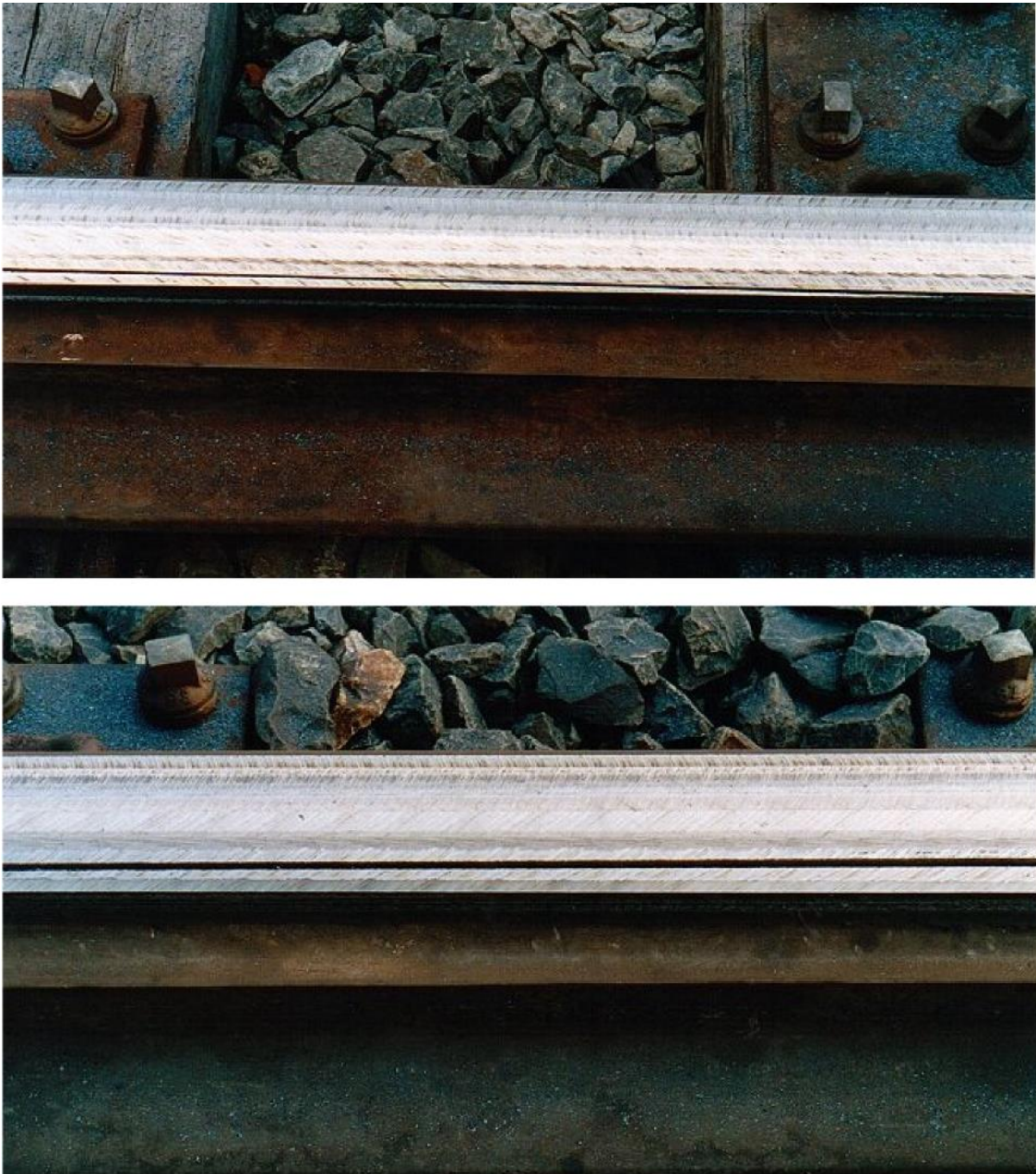
Figure 25 Acceptable Profiling Finish at Switch and Stock Rails
