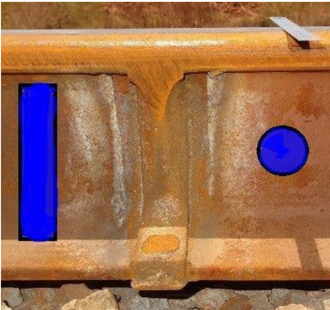
Figure 8-1: Satisfactory Weld quality – Marking example
