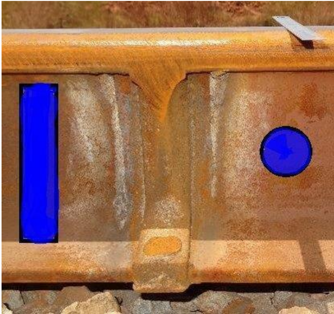
Figure 5: Satisfactory Weld quality – Marking example
