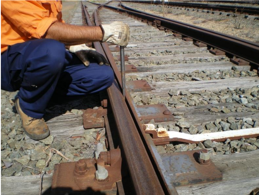
Figure 8-1 Checking tension at manually controlled points
