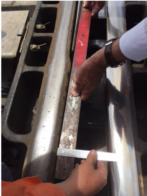
Figure 7-4 Checking protrusion of swing nose crossing
