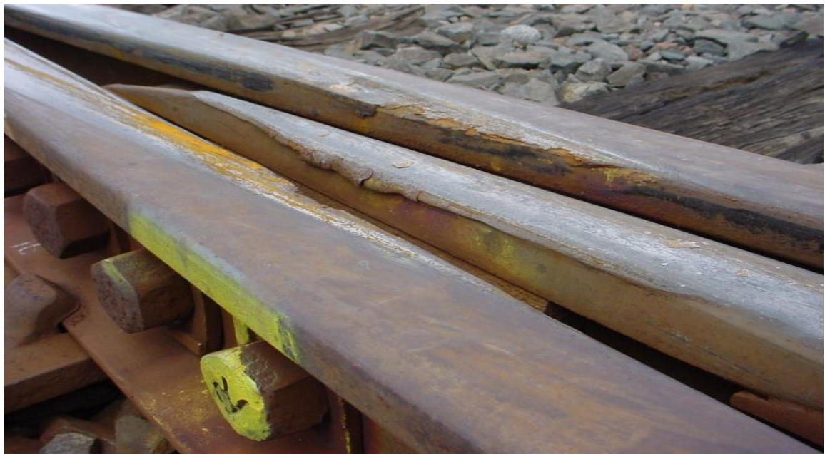
Figure 6-8 Damage to wing rail from wheel transfer
