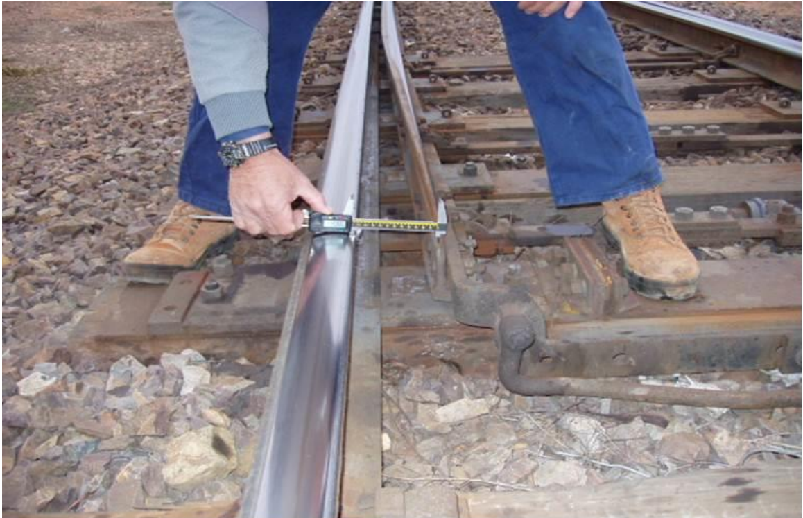
Figure 4-2 Measuring switch opening with callipers
