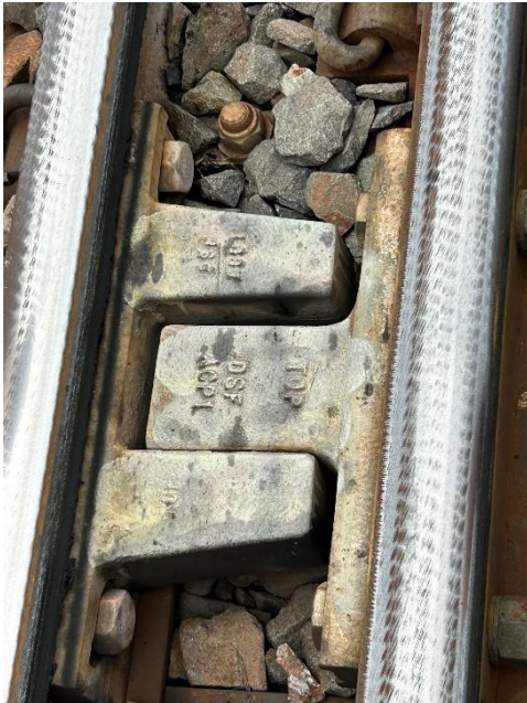
Figure 4-26 Anti Creep Device
