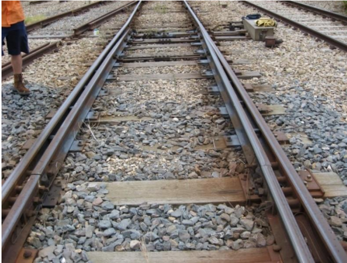
Figure 4-25 Fixed Heel Switch
