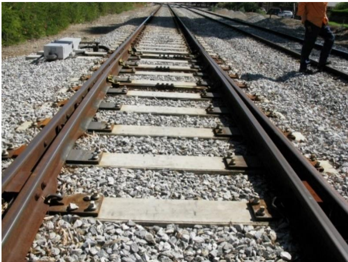
Figure 4-25 Fixed Heel Switch
