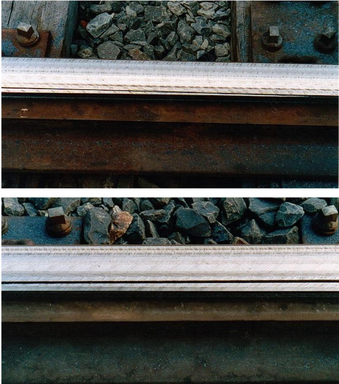
Figure 2 Acceptable Profiling Finish at Switch and Stock Rails
