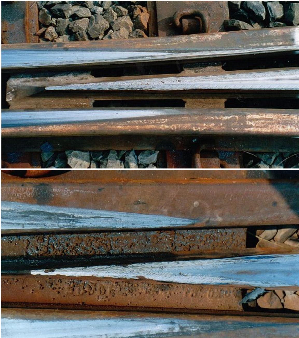
**Figure 3 Acceptable Profiling Near the Nose of V Crossings**
