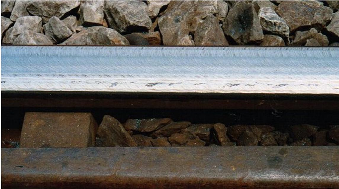
Figure 4 Initial and acceptable residual gauge corner defects before and after profiling
