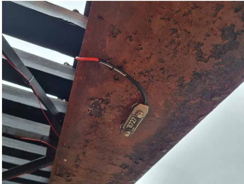
Figure 4-Strain Gauges Installed under the Bottom of the Girders (at Mid-Span)
