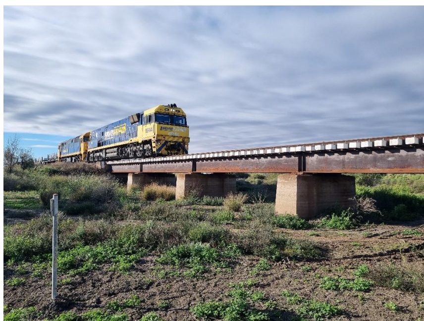
Figure 3-View of the Tested Short Train Crossing the Bridge
