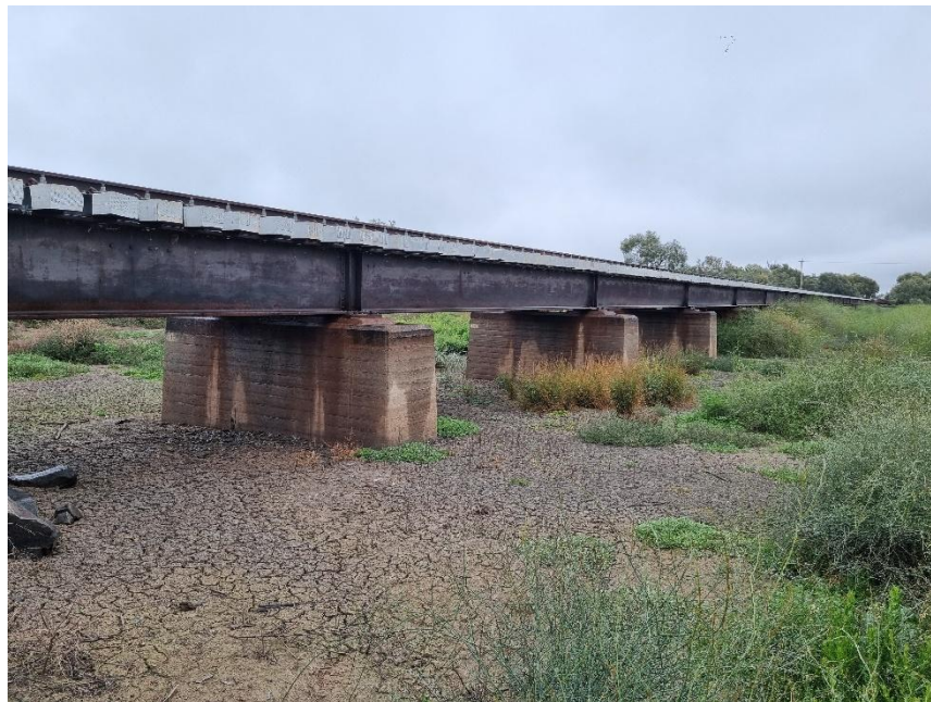
Figure 1-View of the Tested Bridge
