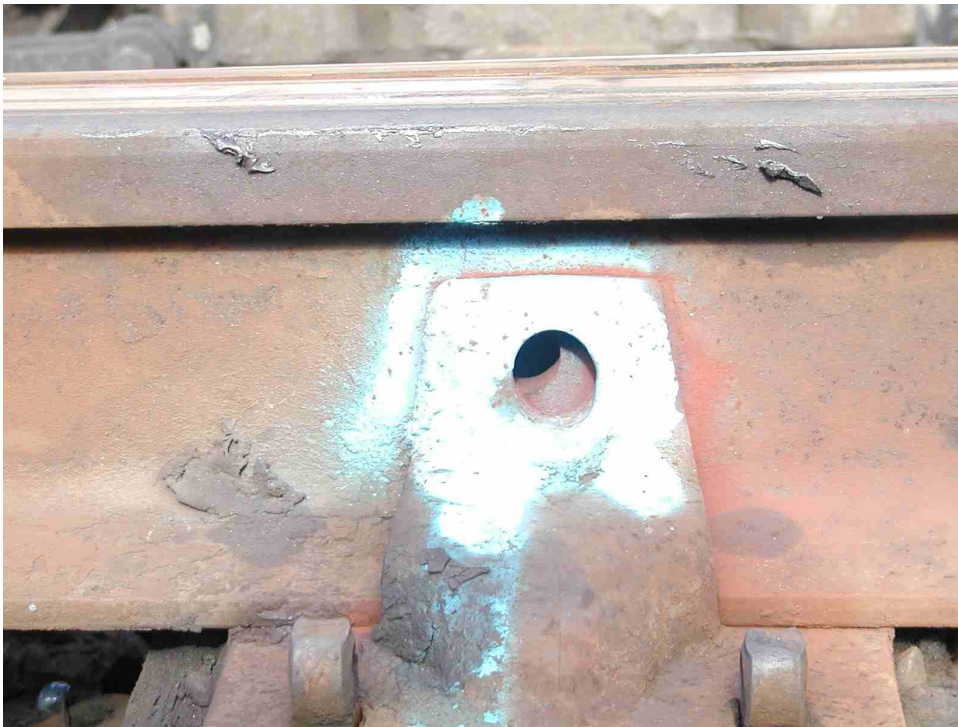
Figure 1 – Mismatched holes
