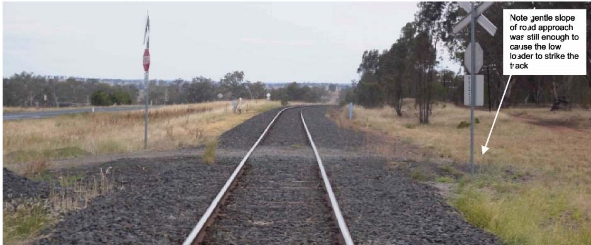
This Level Crossing was, quite reasonably, assessed as being level
