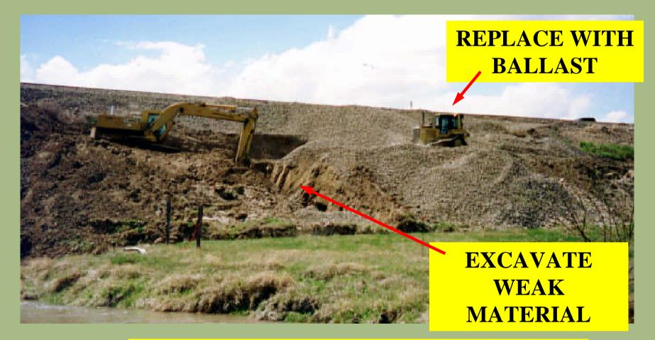
**Replacement performed in short segments under the guidance of a geotechnical engineer**
