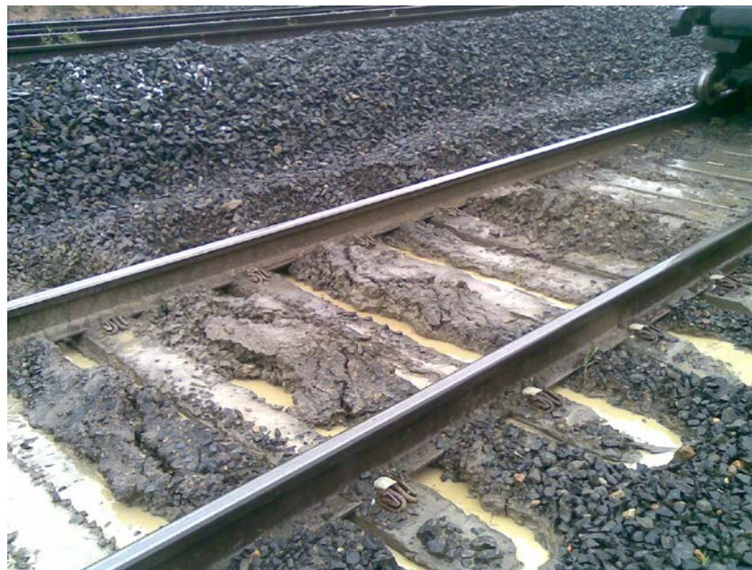
Photo 2.2.1 – Fouled ballast type mud hole (This is a perched type with water and mud in pockets around the sleepers)
