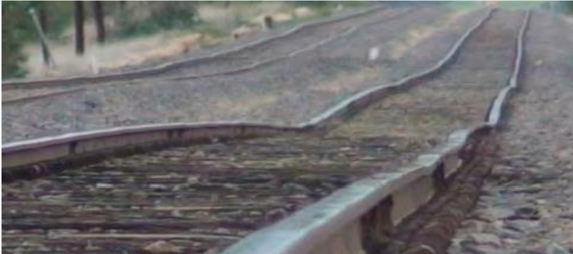
Figure 6: Soft formation mud hole
