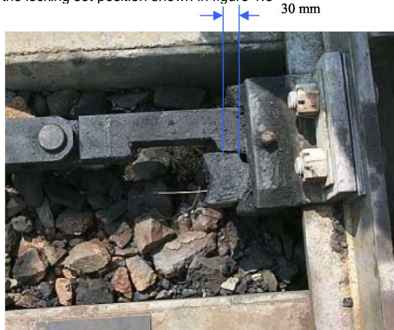
Figure 1.6 – Locking set dimension
