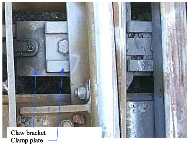
Figure 1.2 – VAE Swing Nose Crossing
