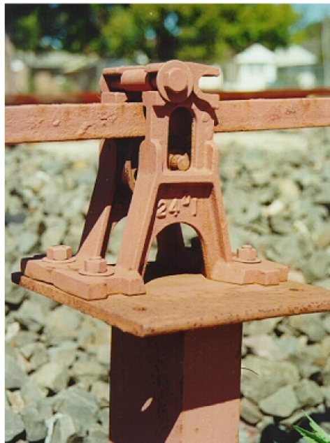
Figure 2.1.5 Channel Rodding A frames and Stands
