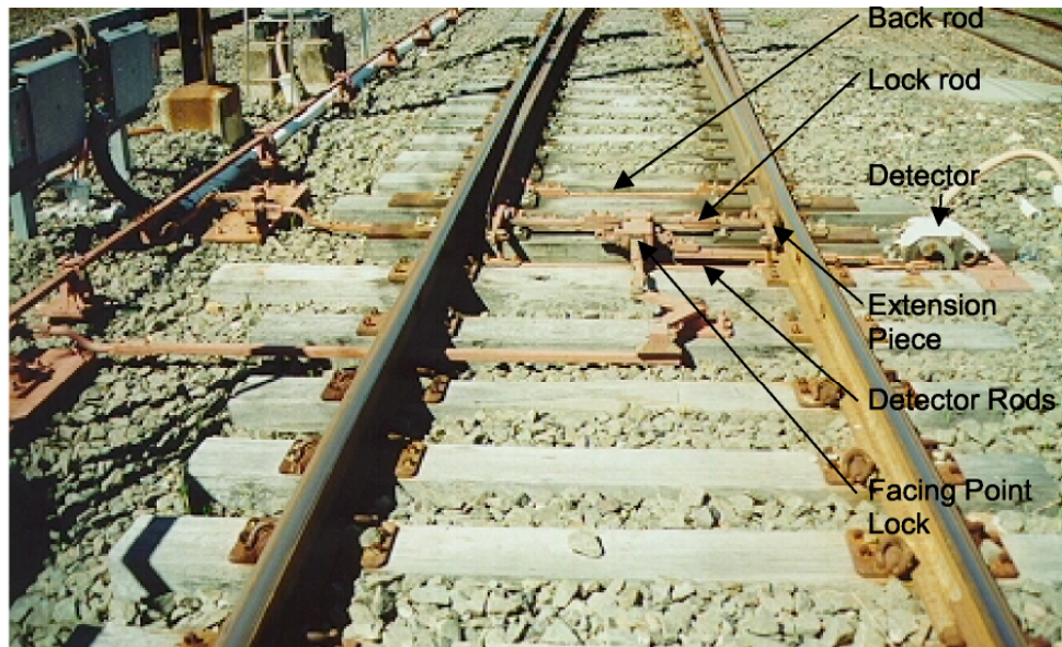
Figure 2.1.11 -Typical Facing Point
