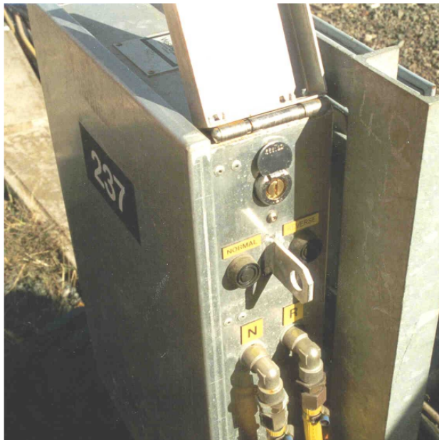
Figure 1.3 - Style S master valve with EOL switch and push-buttons
