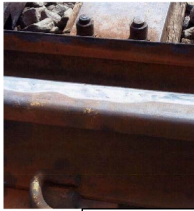
Rail Head Damage
