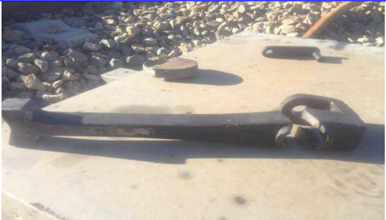
Fig 1. Points were pumping at the B and C timbers, which caused excessive stress and wear causing subsequent failure of the claw (See Above).
