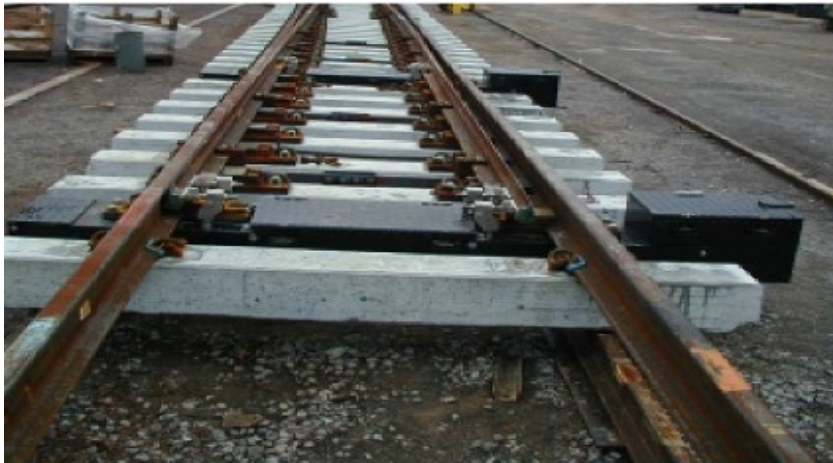
Figure 20 Separate mechanism for front and back drives
