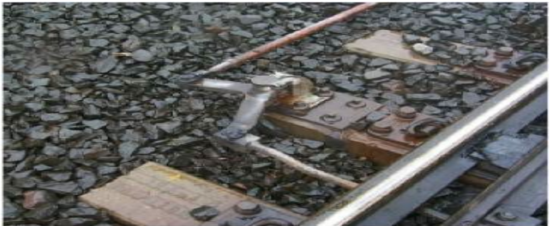
Figure 19 Mechanical back drive
