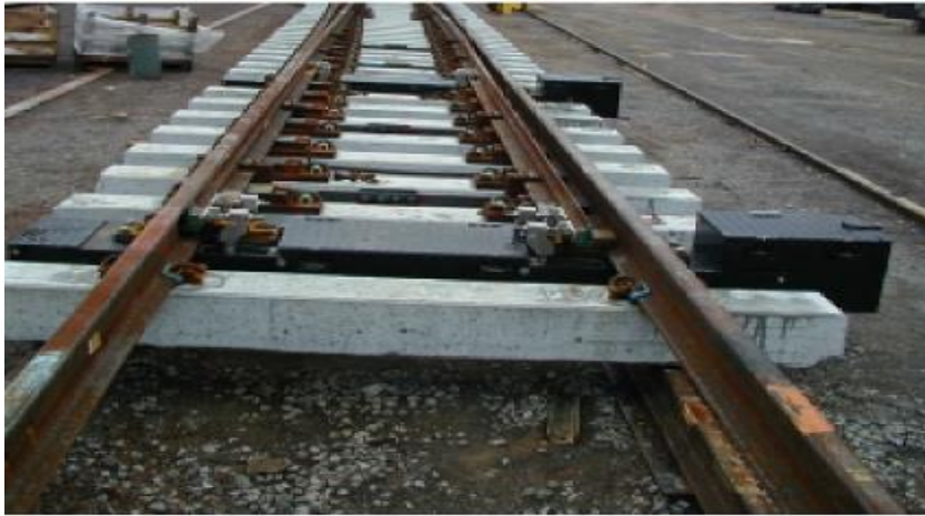
Figure 20 Separate mechanism for front and back drives
