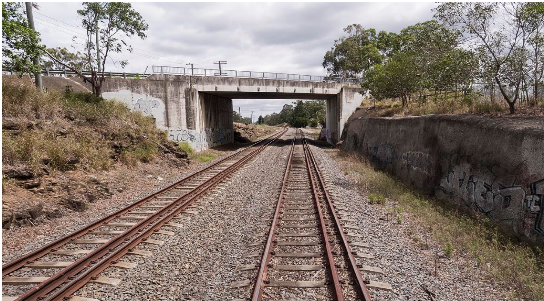
Figure 1 - Typical Dual Gauge Track Arrangement
