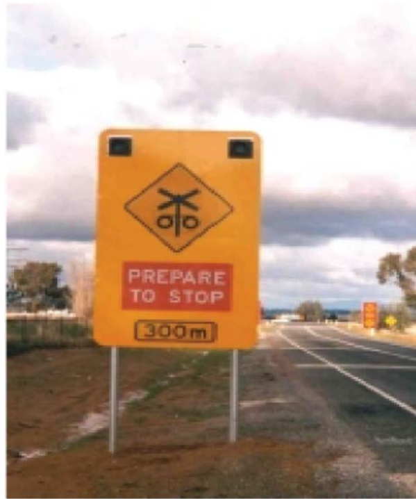
Figure12.2 Advanced warning sign
