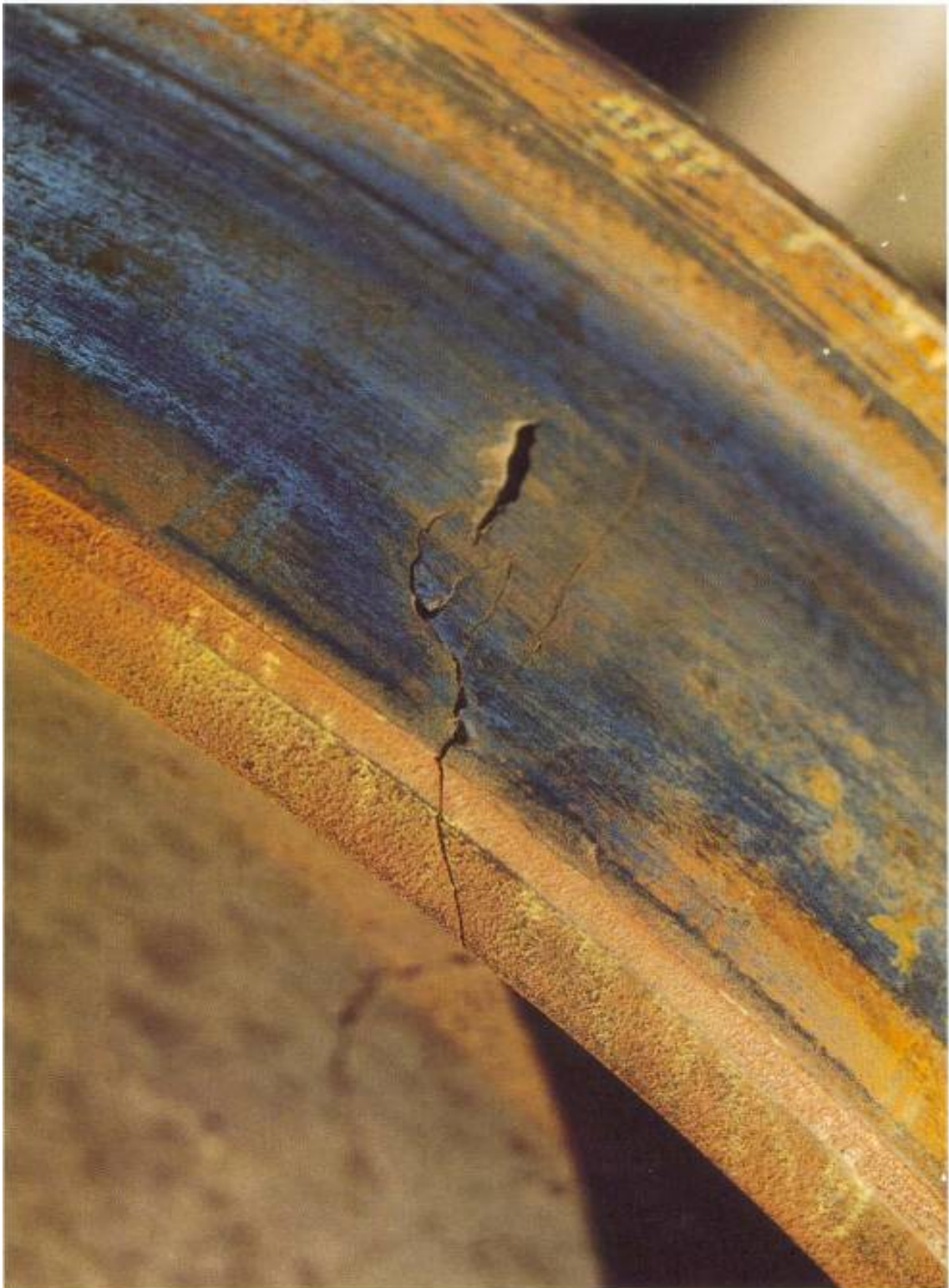
CLASS 5 FATIGUE CRACK
