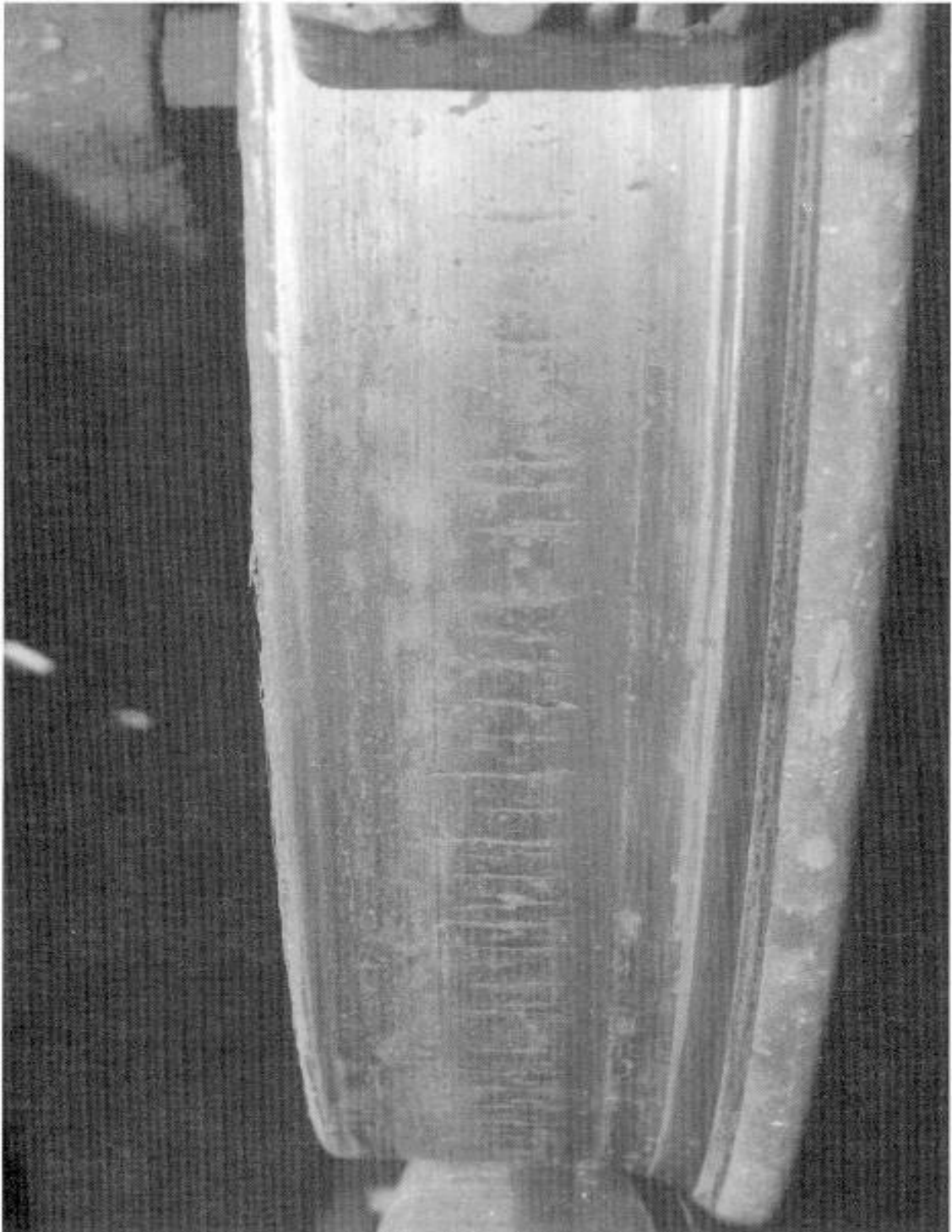
CLASS 2 THERMAL CRACK
