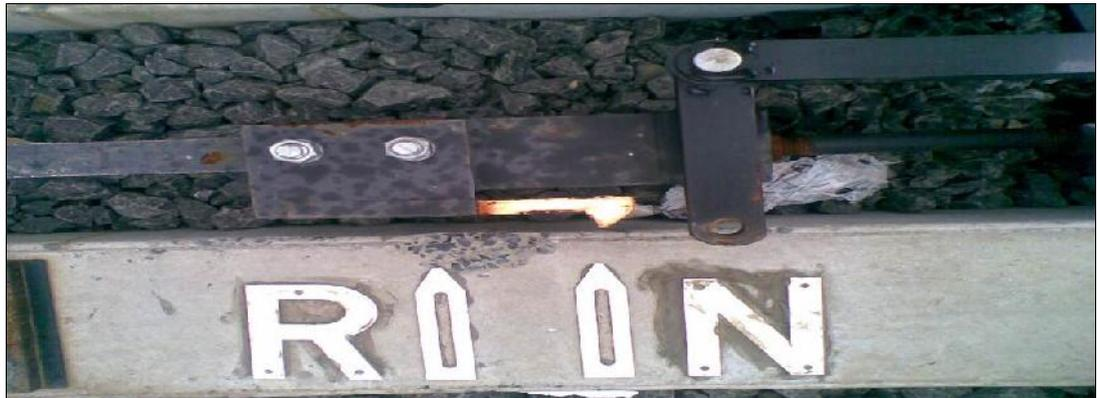
Figure D2 – Example of claw-lock signage
