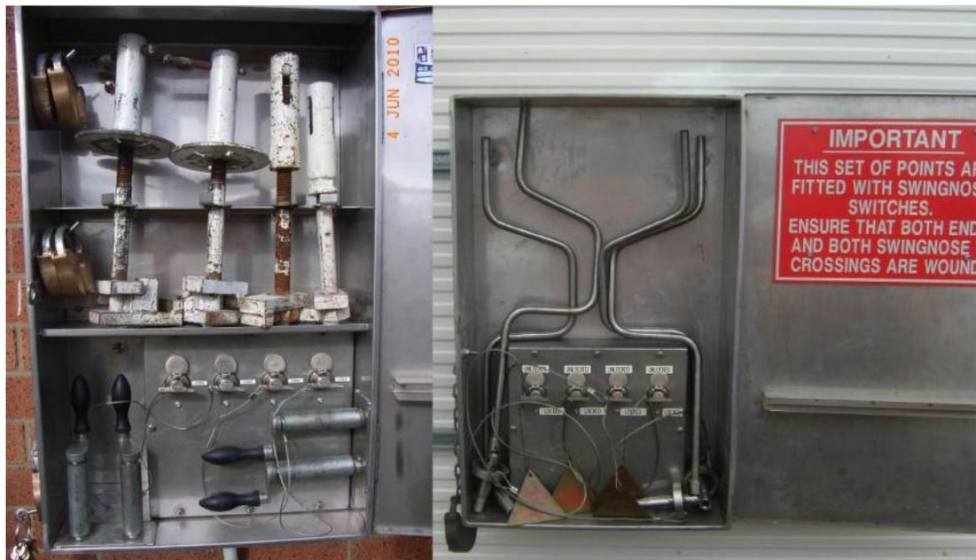
Figure D8 – Typical EOL cabinet for Siemens S700 and Vossloh Cogifer point motors.
