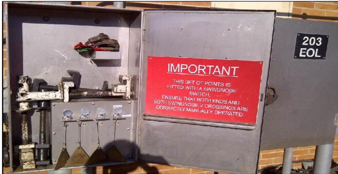
Figure D9 – Typical EOL cabinet for Siemens S700 and Vossloh Cogifer point motors.
